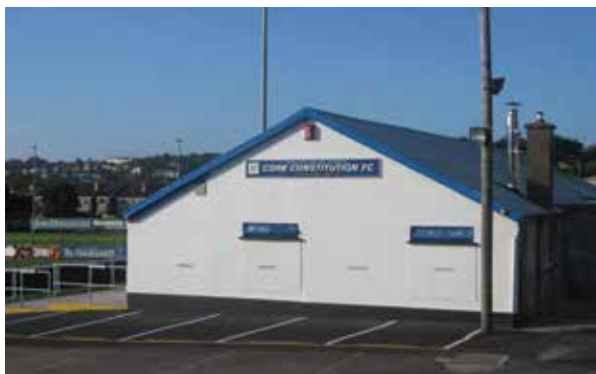
Refurbished Juvenile Dressing Rooms c.2000
