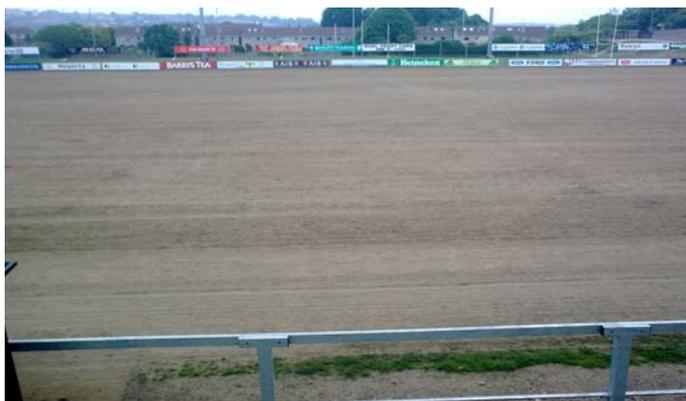
Following this the surface was slit and opened out to a depth of 6 to 8 inch this with 4 inch spacing. This was to aid drainage. The surface was then levelled and the seeding took place. This year a new machine was used to seed the pitch it deep seeded the surface this meant that the seed was laid in tightly packed lines or drills.
