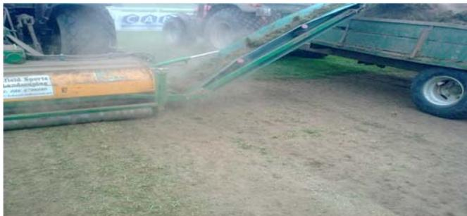
The next stage was to load the surface with 90 tons of course grained sand specially brought in from Rosslare which was spiked into the surface to a depth of 5 inch.
